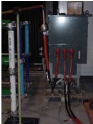
Cold Applied Bushing Boots undergoing successful Impulse testing to 95kV
